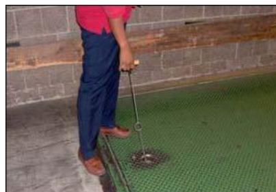
After - Use of a tool allows the dock leveler to be positioned while standing
